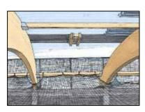
Temporary facilities may include scaffolding, guardrails, safety nets, shoring, falsework, and other forms of temporary support. These need to be planned and designed.
