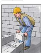
Block lying involves repetitive lifting actions. Lifting dense heavy blocks can cause musculoskeletal problems. The risk of injury can be reduced by specifying alternatives such as smaller or lighter blocks.
