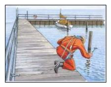
This risk can arise when crossing water to reach a place of work, and when working over or nearby water. These risks can be managed by the provision of suitable systems of work and equipment together with effective means for rescuing and treating workers in the event of an incident.
