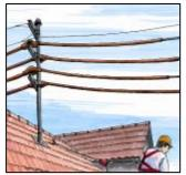
Work near high voltage power lines can cause serious and fatal injuries due to direct contact with live lines or arcing from those lines to nearby plant and equipment. These hazards can be avoided by good design, by making the lines dead for the duration of the work, (clearly the best option), or by effective management controls involving safe working methods and the clear demarcation of zones (in consultation with the line operators) from which plant and machinery should be excluded.
