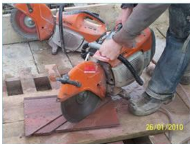
Dobra praksa – rezanje strešnikov z rezalnikom ploščic (National Federation of Roofing Contractors Ltd, GB)
